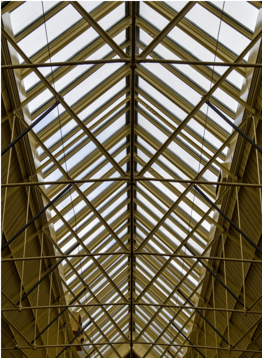
Below: The Station roof
