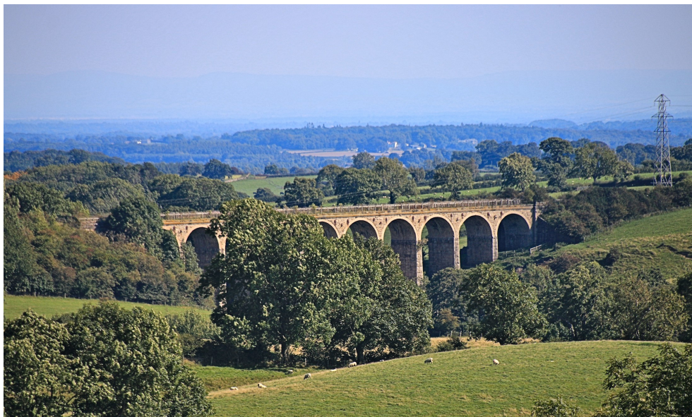
Langley Viaduct - photo by Ian Royston
